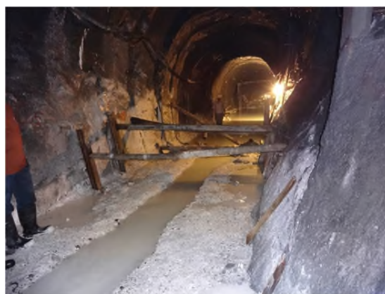
Chamelia Project 50% squeezed headrace tunnel
